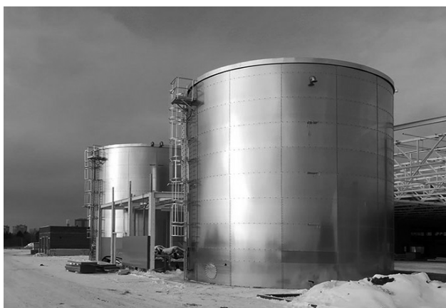
Fig. 1. Vertical steel cylindrical tanks for petroleum products
